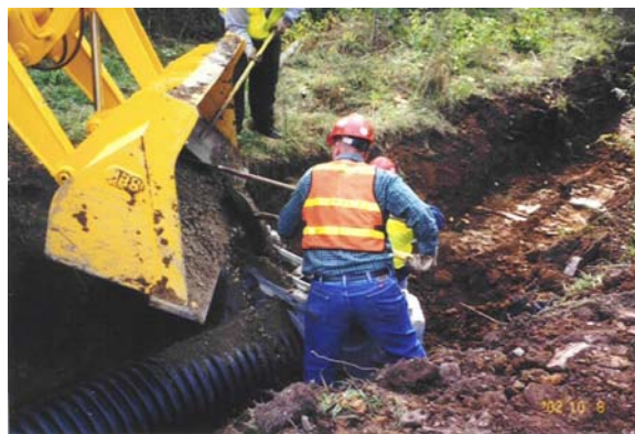
Filling End Wall with Material
