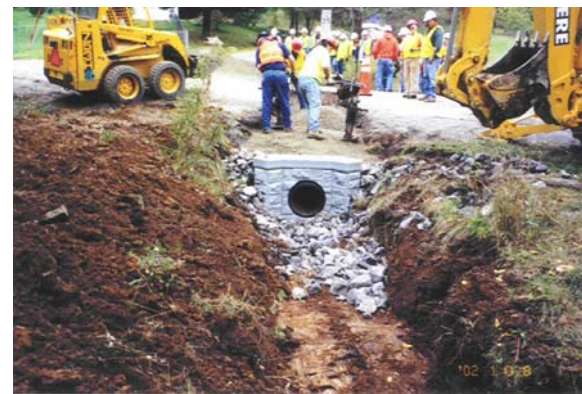
End Wall with Backfill Material Behind It
