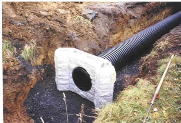
HartmanEW End Wall with Pipe - 1
