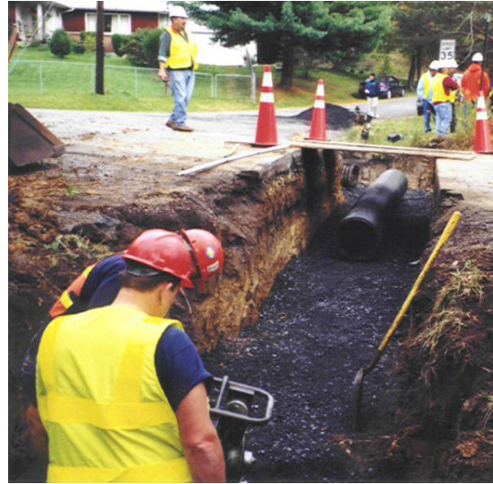
Preparing the Ditch
