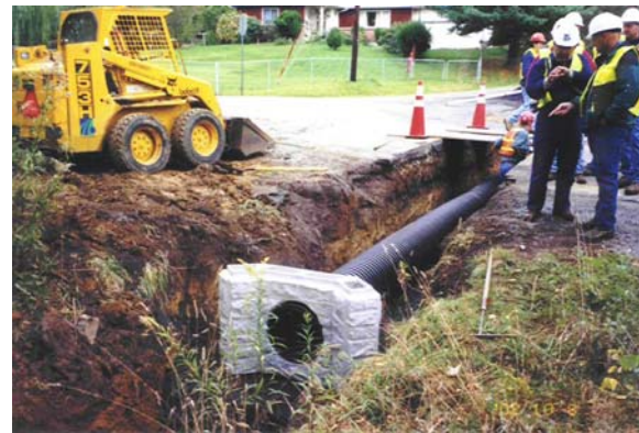
HartmanEW End Wall with Pipe - 2
